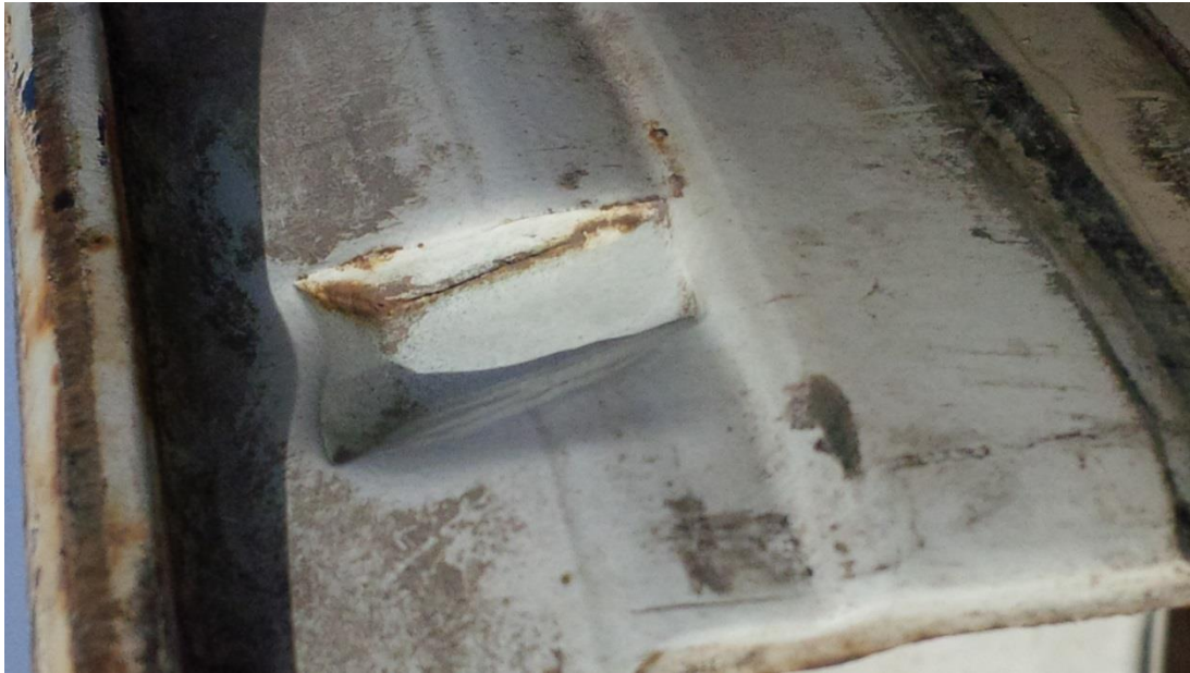
Close up of raised area of the valve stem locator from the bottom (inside) of rim. Cracks in the paint only no damage evident
