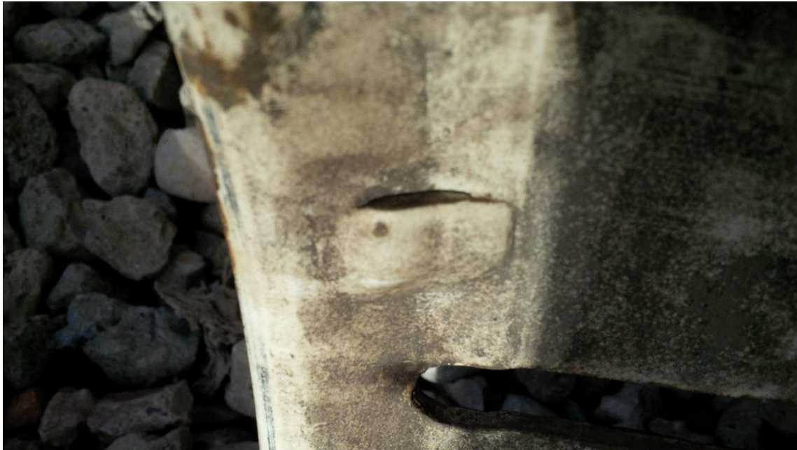
No Damage. Cracks in coating only
